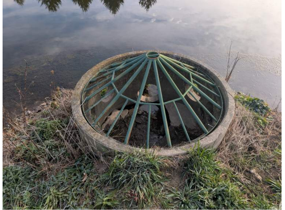
Pond North Outlet Structure
