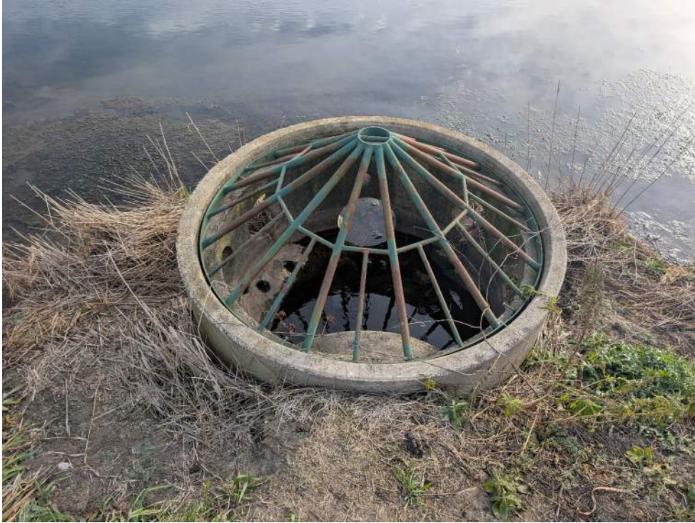
Pond South Outlet Structure
